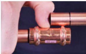
7B. Check the depth mark
