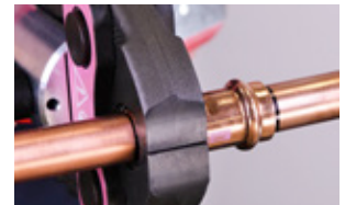
10. Complete the joint with the approved tool. Press once only
